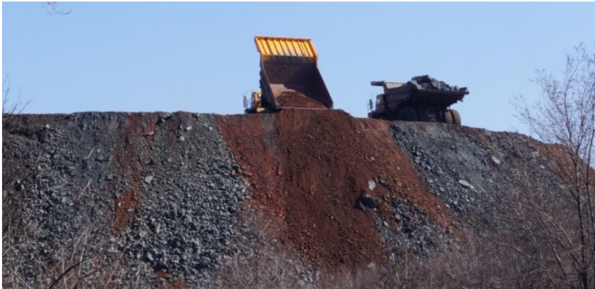
Figure 3 – Construction of a waste dump involving mixed rocks
